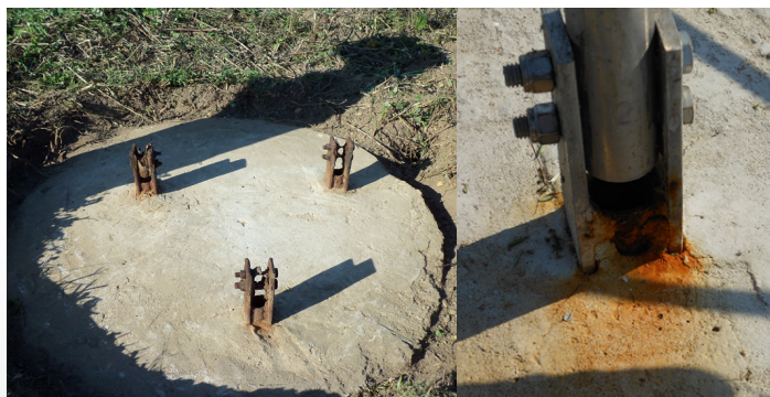
Figure 2: Corrosion in a coastal environment
