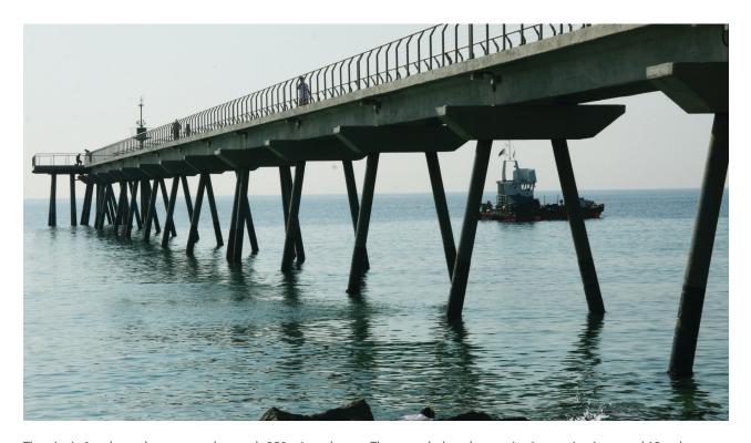
The pier is 6m above the water and extends 250m into the sea. The water below the monitoring station is around 12m deep.
