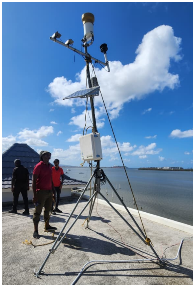
The automated weather station bolted to the roof of the Glistening Waters Hotel
