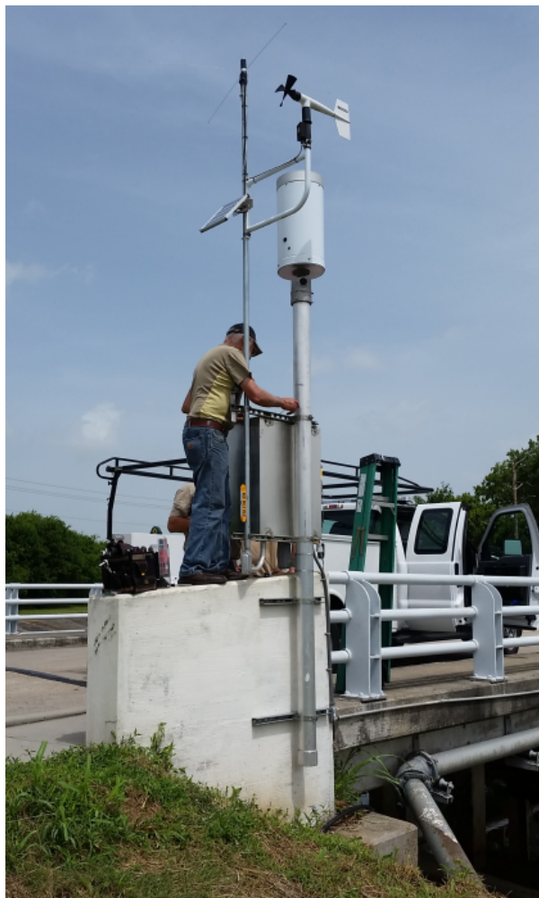
Installing Campbell system for HCFCD
