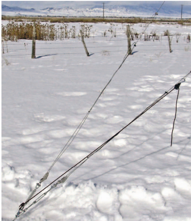
FIGURE 2.4-8. Rope Ratchet Assists Assembly
