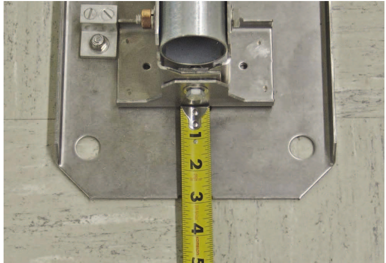
FIGURE 2.4-1. Tape Measure in Slot for South Anchor
