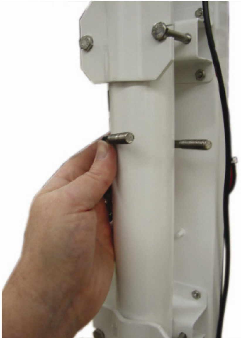
FIGURE 2.5-9. Slide Antenna Bracket U-Bolt around Back of the Pole
