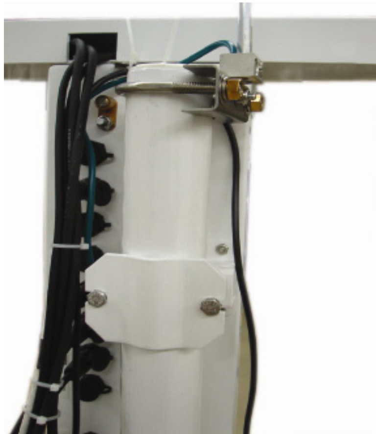
FIGURE 2.5-8. Loosely Drape Antenna Cable over Back of Enclosure
