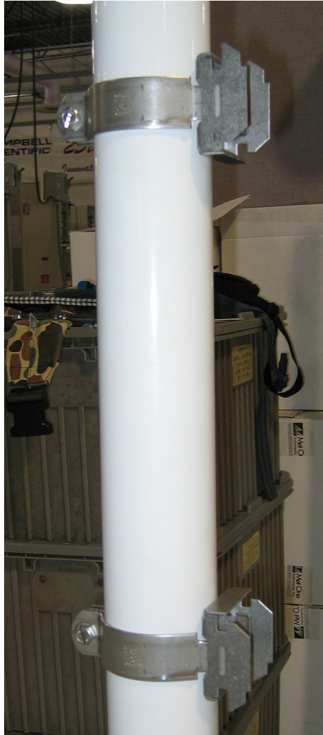
FIGURE B.2-2. Both Strut Clamps and Brackets on T107 Pole
