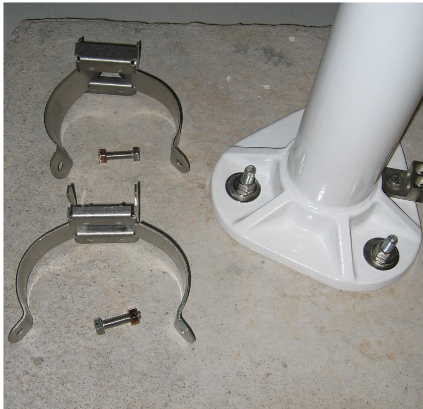
FIGURE B.2-1. Strut Clamps in Brackets
