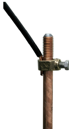
FIGURE 2-14. The #4 cable connected to the ground rod.
