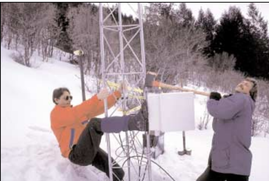
Intrepid Campbell Scientific employees install a meteorological tower in preparation for Salt Lake City's Olympic Winter Games bid (winter 1990/91).
