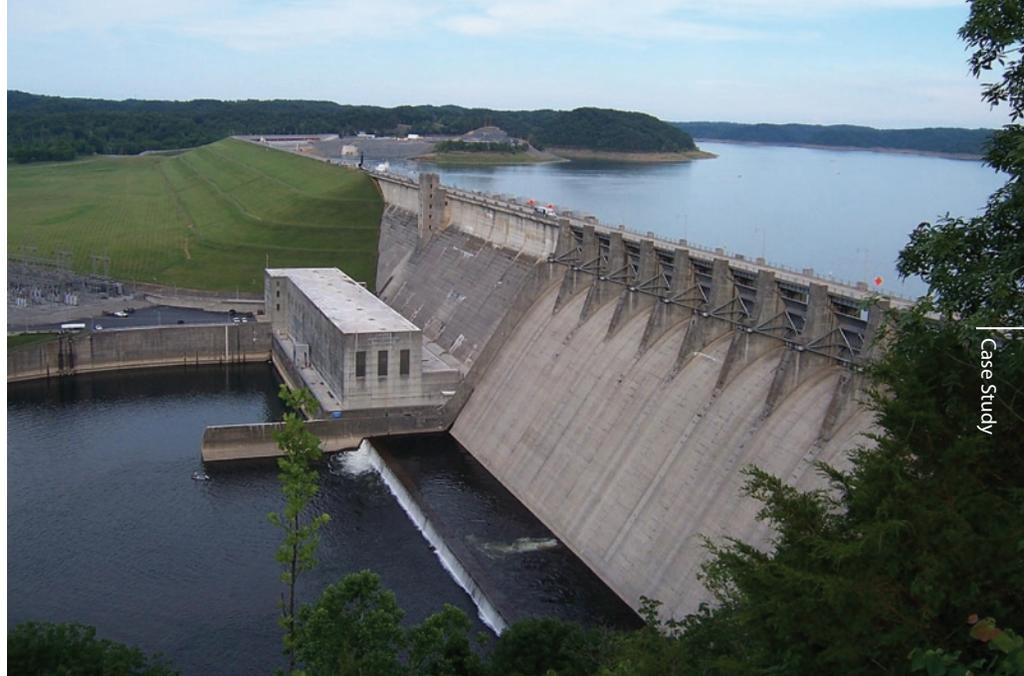
program to be followed by construction of a nearly 1,000,000-square-foot concrete diaphragm wall. As part of the monitoring and analysis portion of the project, the Army Corps of Engineers (USACE) retained URS Corporation to design, install, and operate an automated data acquisition system (ADAS). The ADAS monitors the large number of piezometers measuring water level (seepage from the reservoir) in the embankment.
