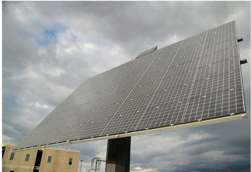
a stationary station with a reference solar panel, and then instrumented that reference station and the tracking solar array with temperature sensors, pyranometers, and power-output sensors. We will be able to measure the output of a panel on the tracker tower and compare it to the
