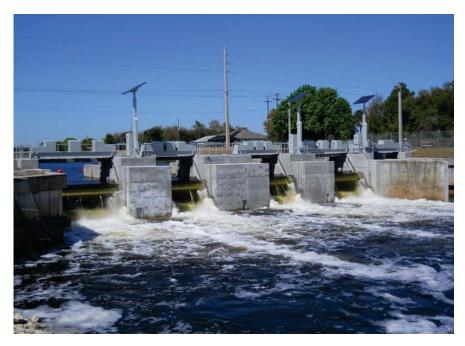
SJRWMD offices, and is also installed on a SJRWMD laptop computer, giving managers the flexibility to control the gates from any location. Two cameras are positioned to view the gates. They interface with the dataloggers and software to enable remote viewing of the site.
