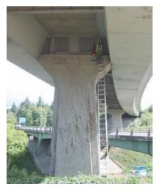
Kamal's Bridge in Tualatin is a steel boxgirder bridge with four spans crossing Interstate 5. ODOT sought to improve the monitoring of the bridge's structural response to changes in temperature and traffic load. This was needed because fatigue cracking appeared between the transverse cross beams and the longitudinal box girders on either side of the bridge deck.
