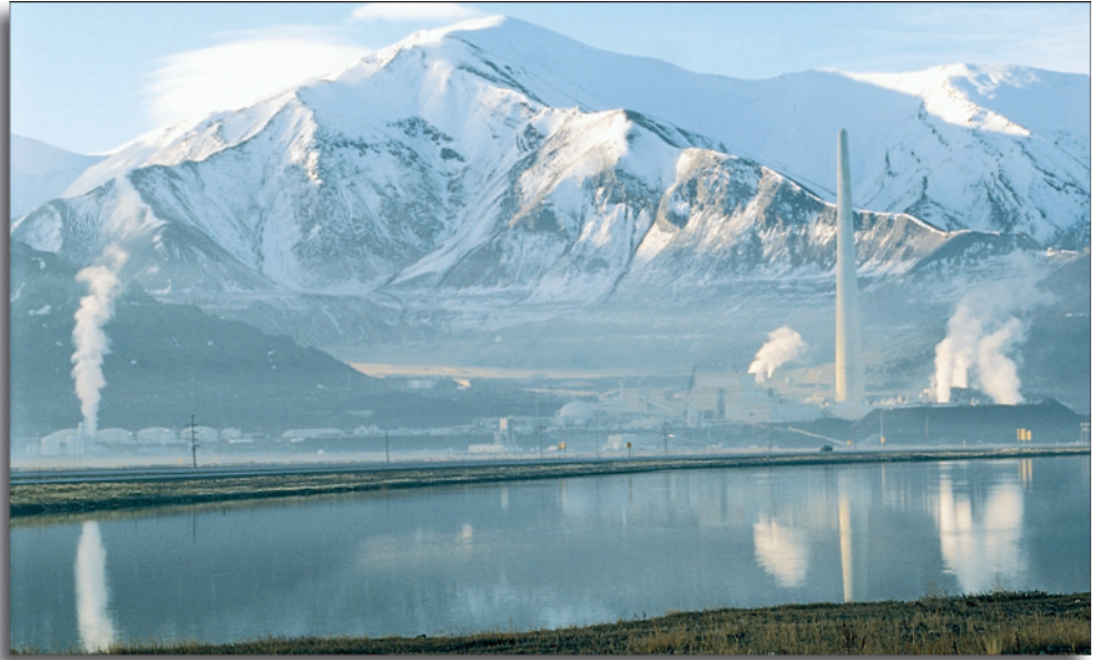
Gas and particulate concentrations, as well as meteorological conditions that affect air quality, can be monitored locally and regionally with a network of stations.
