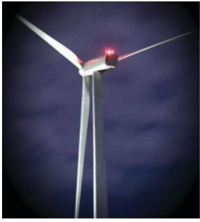
Aircraft warning light intensity controlled automatically by visibility sensor
