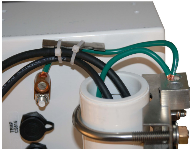
FIGURE 2-40. Grounding to Lightning Rod Clamp
