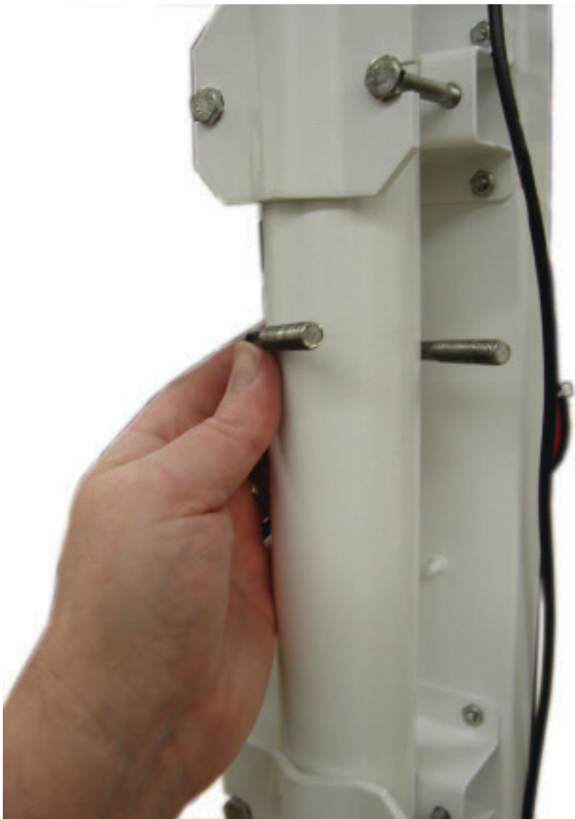
FIGURE 2-31. Slide Antenna Bracket U-Bolt around Back of the Pole
