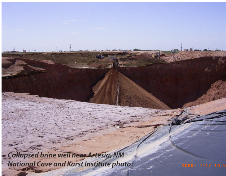
Collapsed brine well near Artesia, NM National Cave and Karst Institute photo
