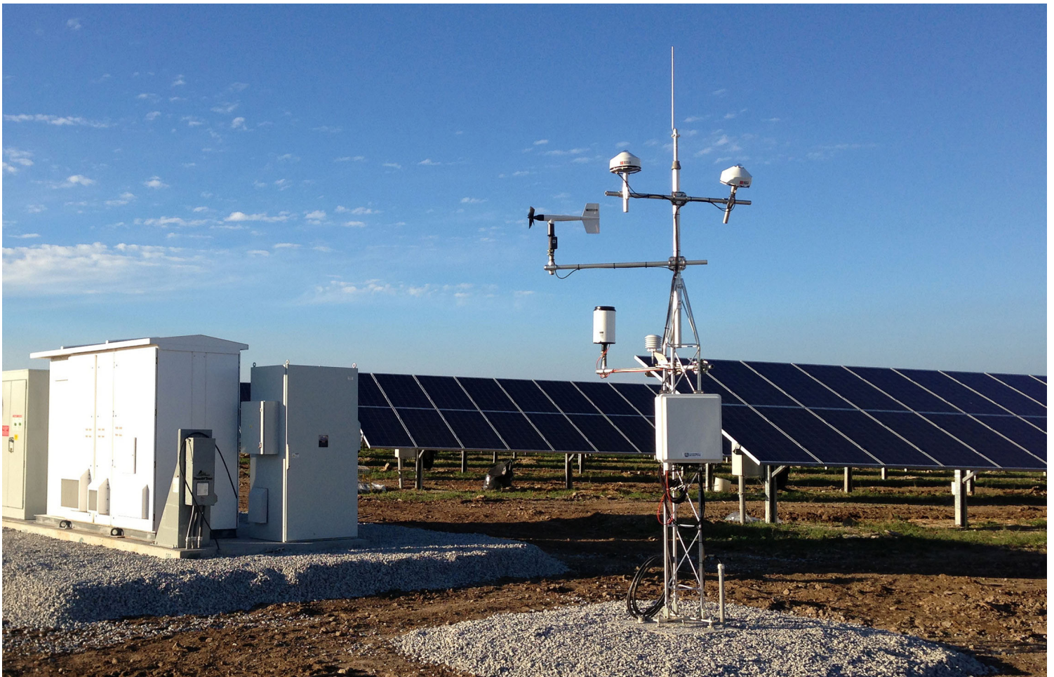
An automated weather station for solar-farm performance monitoring. This turn-key system was customized by Campbell Scientific to meet the specific requirements for Ontario solar farms.
