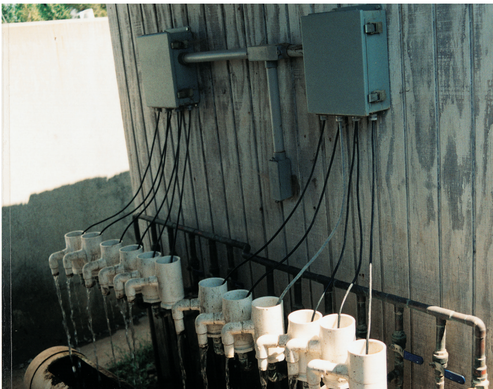
Rather than deal with the added expense of extra cable lengths for 12 individual dissolved oxygen probes, Stolt Sea Farm devised a system in which water continuously flows from the tanks through PVC pipe to sensors at the monitoring station.
