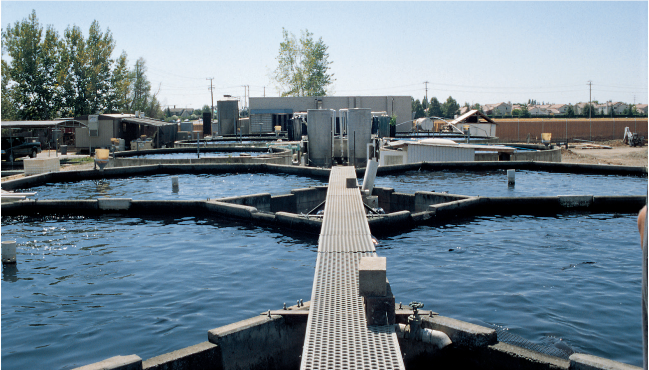
A Campbell Scientific system continually monitors and controls water quality in each of 12 individual tanks at the Stolt Sea Farm facility in Elk Grove, California. The tanks house sturgeon, raised to produce premium caviar.
