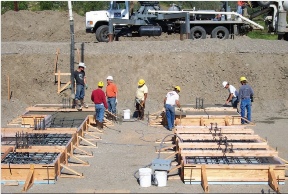
Monitoring concrete curing and the affect of the insulation.
