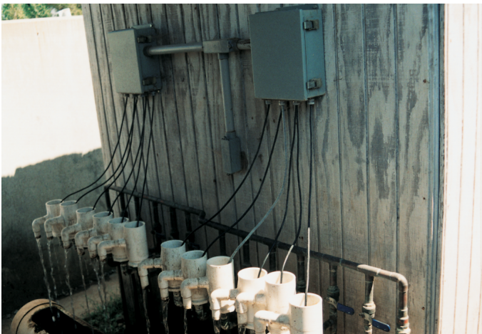
Rather than deal with the added expense of extra cable lengths for 12 individual dissolved oxygen probes, Stolt Sea Farm devised a system in which water continuously flows from the tanks through PVC pipe to sensors at the monitoring station.
