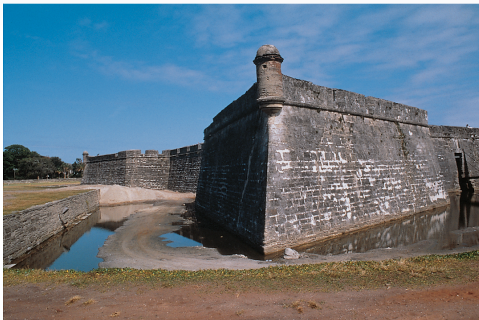
Castillo de San Marcos National Monument, St. Augustine, Florida. Taken in 1995, this view looks across the moat toward the southwest bastion, where several major cracks are visible.
