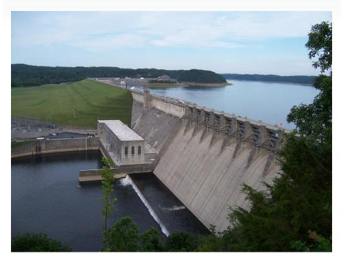
The Wolf Creek Dam near Jamestown, Kentucky, was constructed partially as a regular concrete hydroelectric dam, but mostly as an earth-fill embankment structure. Finished in 1950, within 20 years it developed serious reservoir seepage problems. Several repair projects had a degree of success at stemming the flow, but in recent years managers decided that resurging seepage at the dam constituted an emergency situation.
