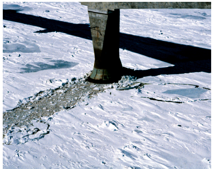
The force of ice floes impacting the bridge and the bridge's response to the impacts are monitored by two CR9000 systems. (Photo courtesy of Boily)
