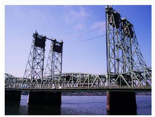
The Oregon Department of Transportation (ODOT), as part of its statewide structural health monitoring (SHM) program, wanted to improve its monitoring of the Interstate 5 Bridge near Portland—a steel bridge approximately 3,500 feet in length with 16 spans. ODOT was particularly interested in the southbound portion of the bridge, which conducts traffic from Washington into Oregon over the Columbia River.
