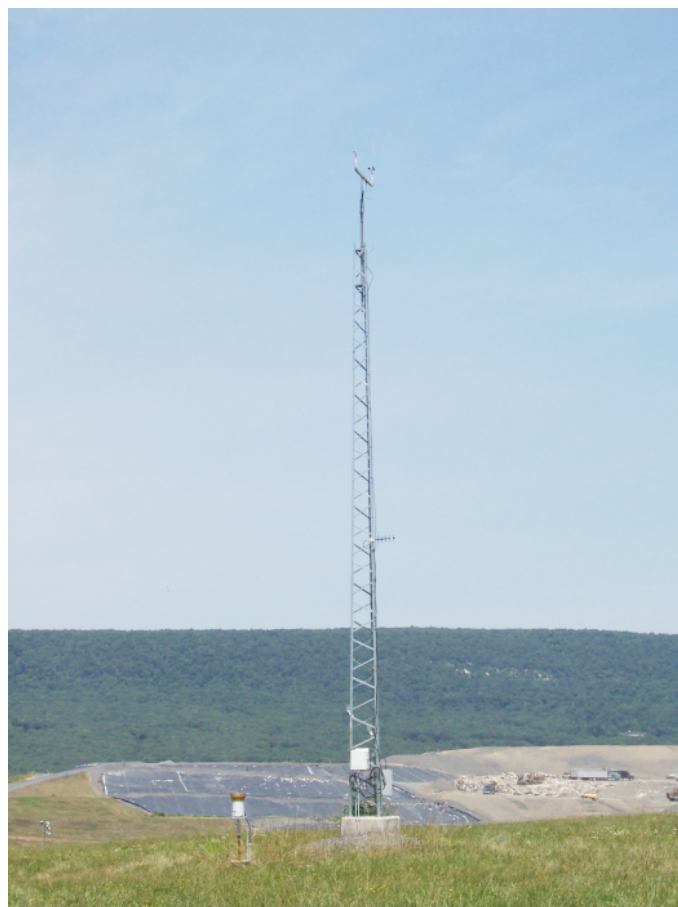
This meteorological tower transmits landfill site conditions via radio. (Photo courtesy of Robert Karpovich)
