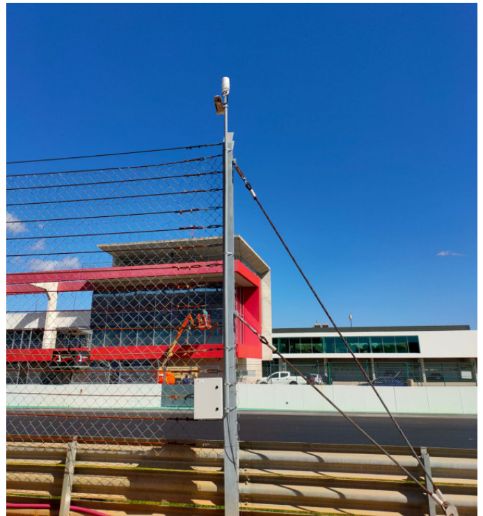
Installation of the weather monitoring system
