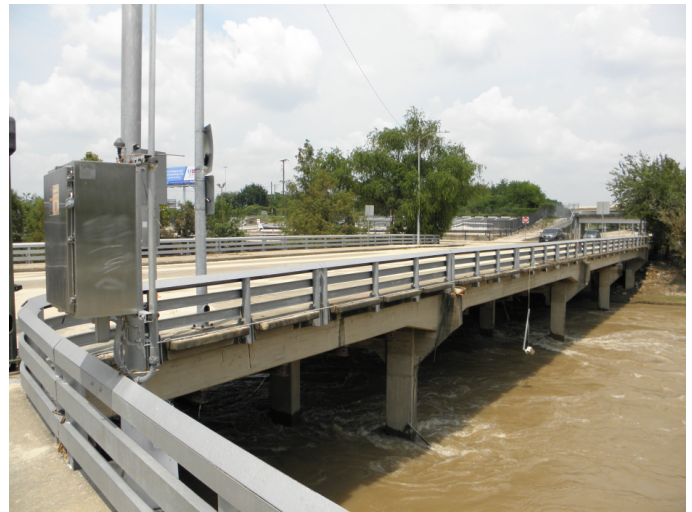
High water from Hurricane Harvey
