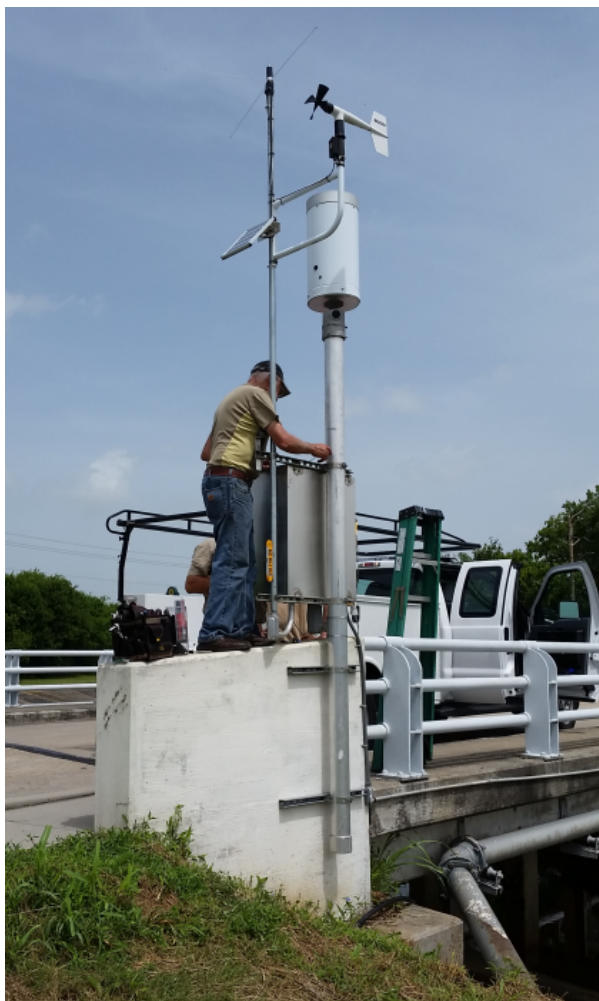
Installing Campbell system for HCFCD
