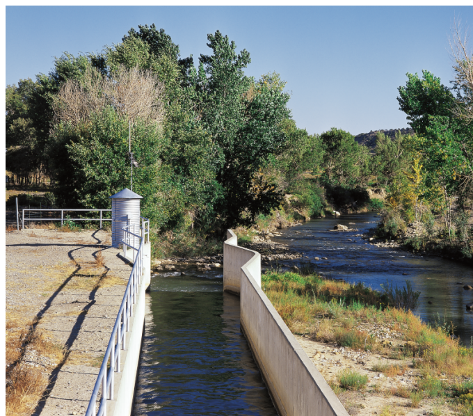
A Campbell Scientific CR10 and a shaft encoder measure return flow to Cottonwood Creek at Swasey Diversion.
