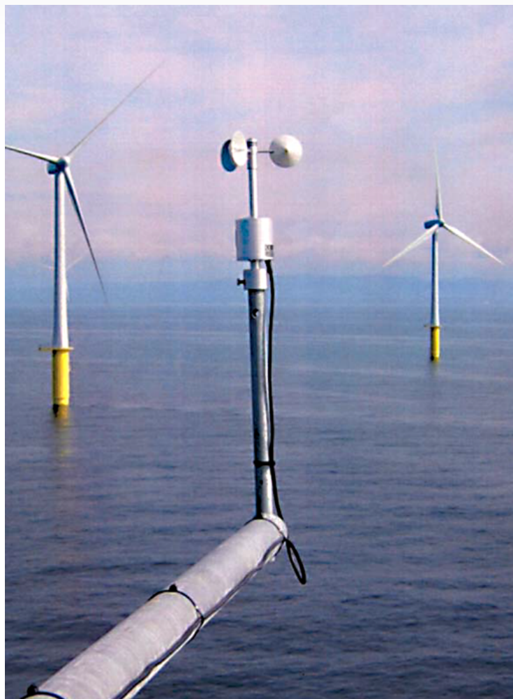
View from one of the anemometers on the meteorological tower to the monopiles and turbines of the wind farm (Photo courtesy of npower renewables)
