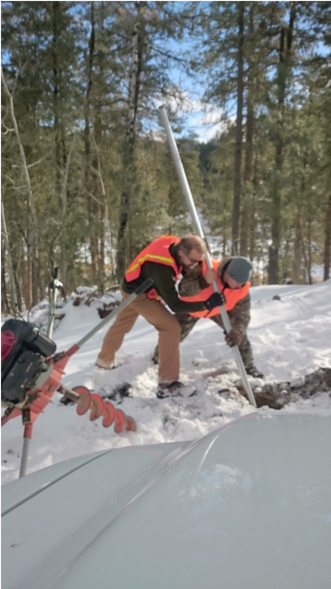
Winter installation of support structure for instrument housing and equipment
