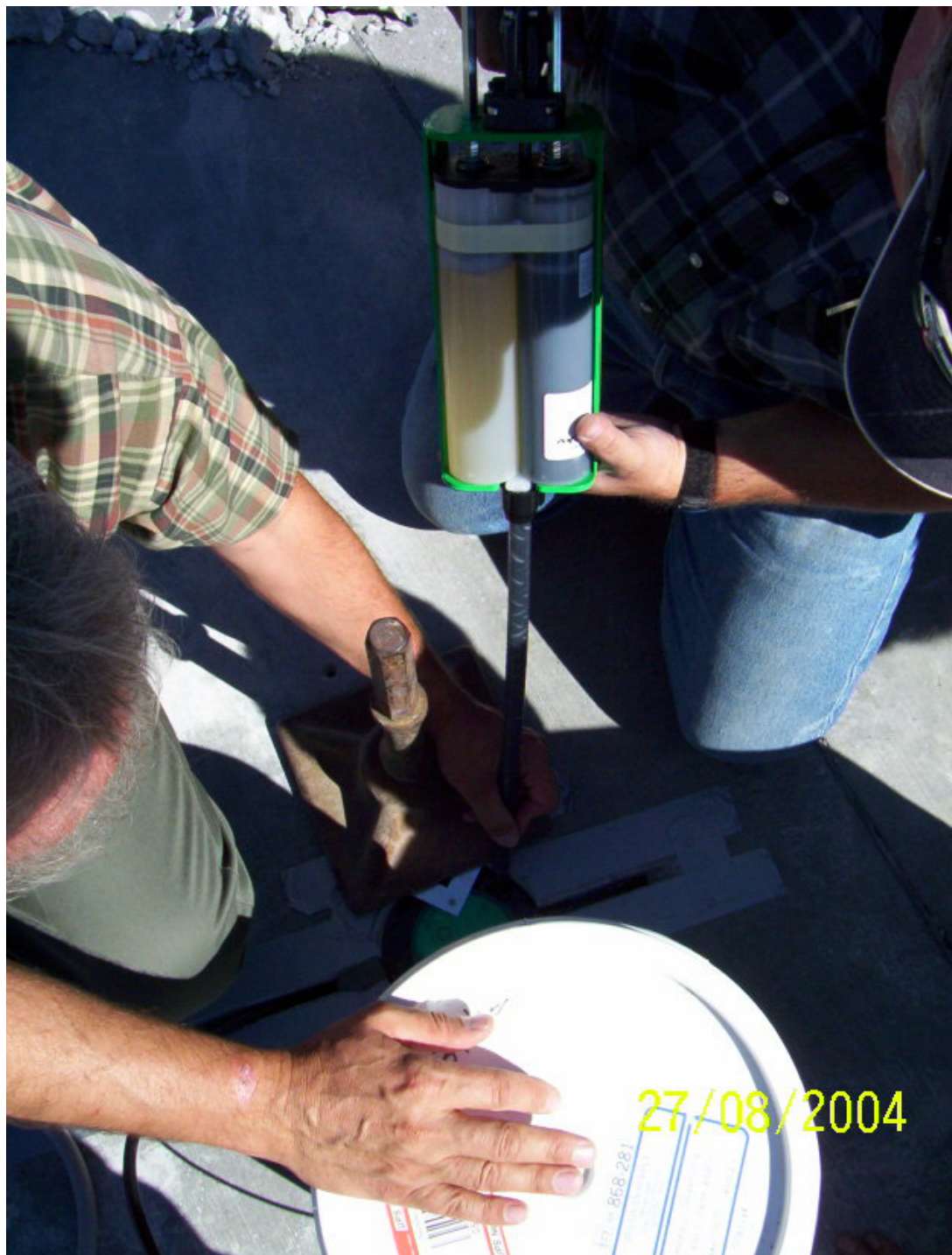
FIGURE 3-6. First pour of Fabick epoxy, pn FJS (fast set), useable between 20° to 180°F.
