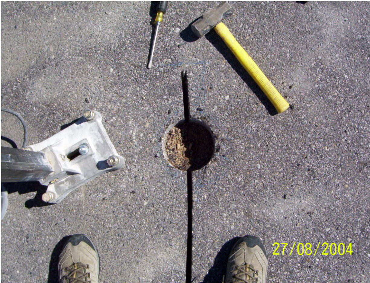
FIGURE 3-1. Core cut for the road sensor.
