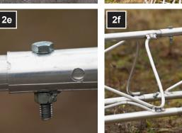
2. Align the top two tower sections end to end in line with the tower base. Connect the sections together, and tighten.
