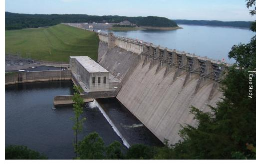
program to be followed by construction of a nearly 1,000,000-square-foot concrete diaphragm wall. As part of the monitoring and analysis portion of the project, the Army Corps of Engineers (USACE) retained URS Corporation to design, install, and operate an automated data acquisition system (ADAS). The ADAS monitors the large number of piezometers measuring water level (seepage from the reservoir) in the embankment.
