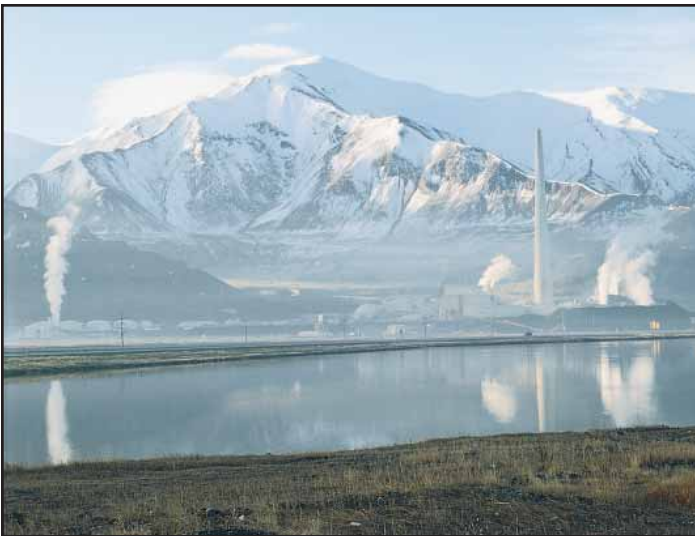
Network of approximately 20 stations continuously monitors air quality, northern Oquirrh Mountains, Utah.
