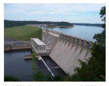
Campbell Scientific equipment monitors seepage at the Wolf Creek Dam. The dam consists of a concrete hydroelectric dam and an earth-filled embankment structure.
