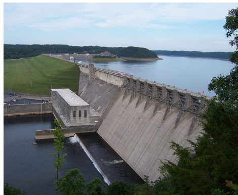
Seepage is monitored for a concrete/earthen dam ( www.campbellsci.com/wolf-creek )
