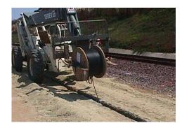
In Del Mar, California, a tractor-mounted trencher installed coaxial cable for monitoring slope stability using our TDR system.
