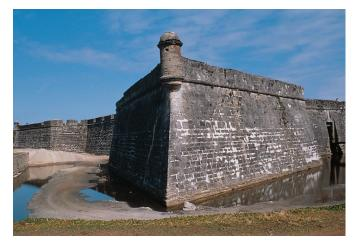
Long-term monitoring at the Castillo de San Marcos is used to determine the cause of cracks in the walls of the 17th century fort.
